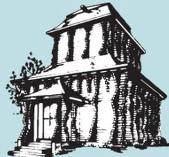
**9. REDWOOD BUILDING** – During the depression, my brother and I hired plenty of workers to erect this one-of-a-kind showplace. It is made from California redwood shipped through the Panama Canal. We used just horizontal 4' x 6' timbers, galvanized dowels instead of nails, and glass block in place of windows. Visiting architects came to gawk.
